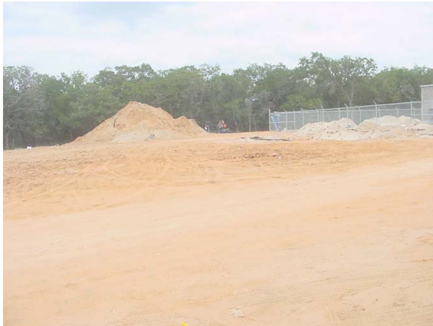
Photo 4 – Approximate bore location B-2 (Nockenut Road Site)
